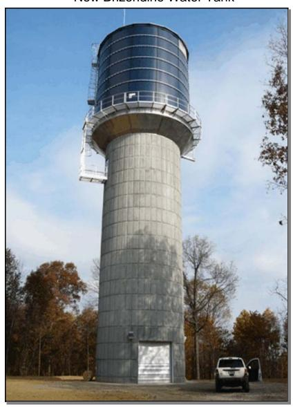
The new 220,000 gallon Brizendine Tank is made of concrete, aluminum and glass lined steel. It will never need painting. This is the first tank of this type built in Kentucky.
